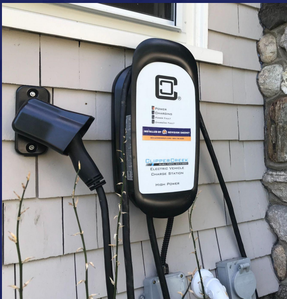
Level 2 charger installed in an 1896 Bath home.
