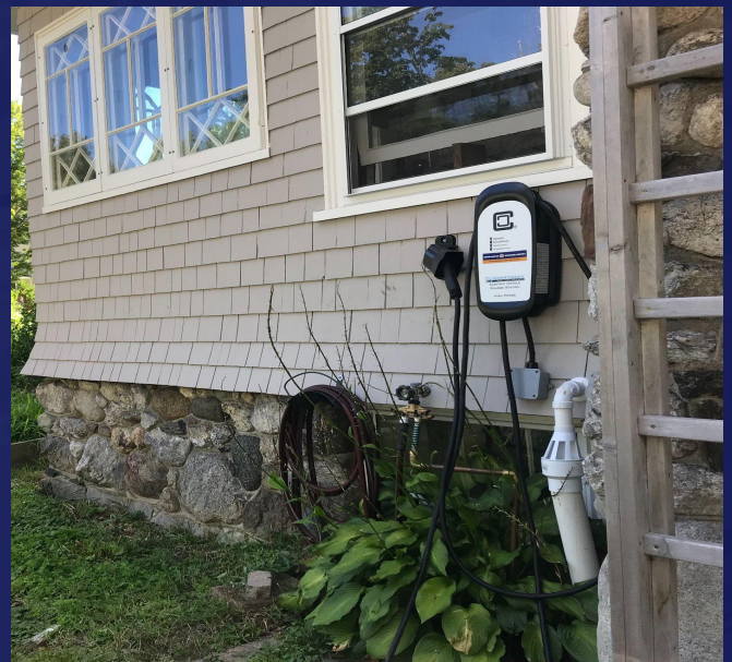
Level 2 charger installed in an 1896 Bath home.
